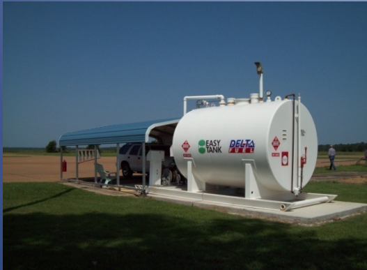
Aviation Fuel Storage Tank
