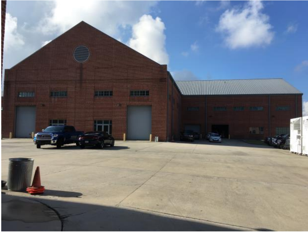
S15886 136004-53; 139 TH RSG READINESS CENTER (REAR VIEW-RIGHT SIDE)
